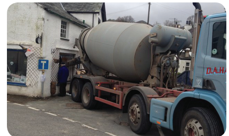
Cement being poured into the shop.
